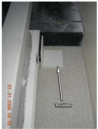
Figure 12: Snubber installed at end of inertia base to restrict lateral movement.
