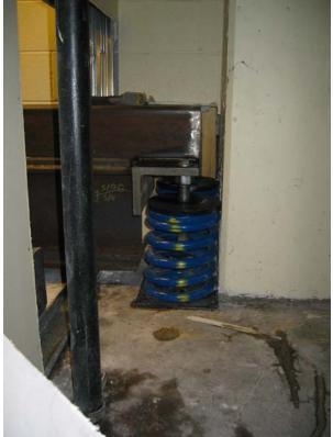
Figure 10: Spring isolator at rear of base at column.
