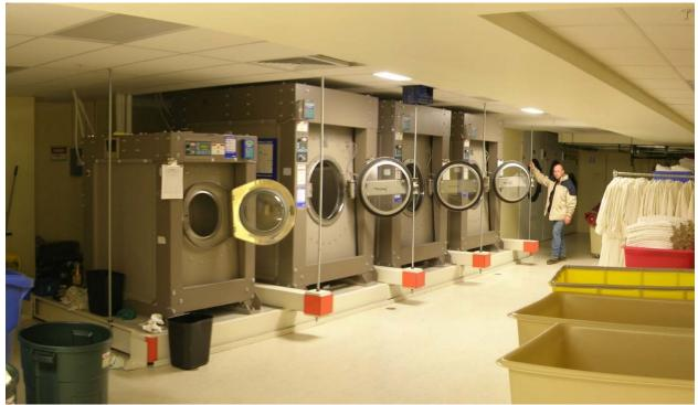
Figure 13: Washer/extractors on retrofitted inertia base.
