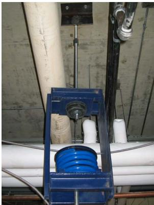
Figure 9: Isolation hanger at front of inertia base.
